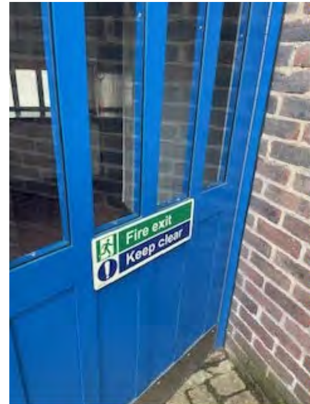
Fire door with fire exit sign at 23-34 Primrose Hill Court.
