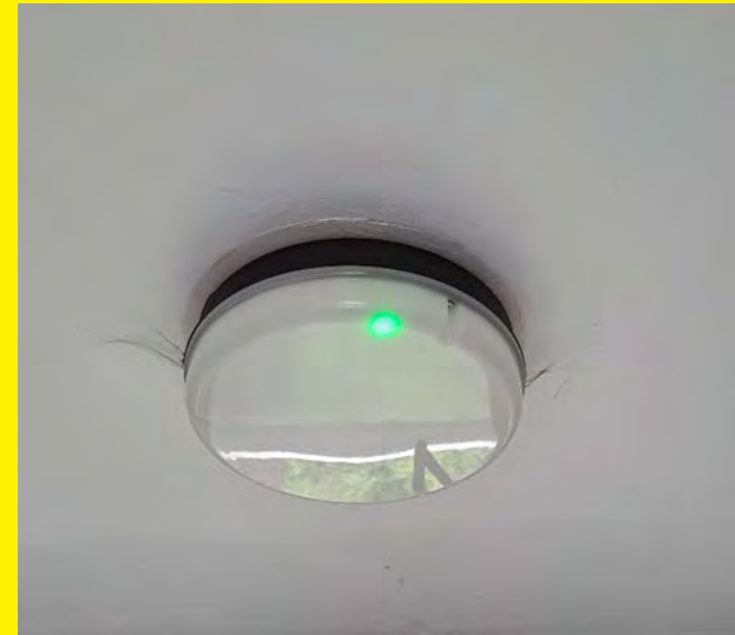
Emergency Lighting at Palgrave House.
