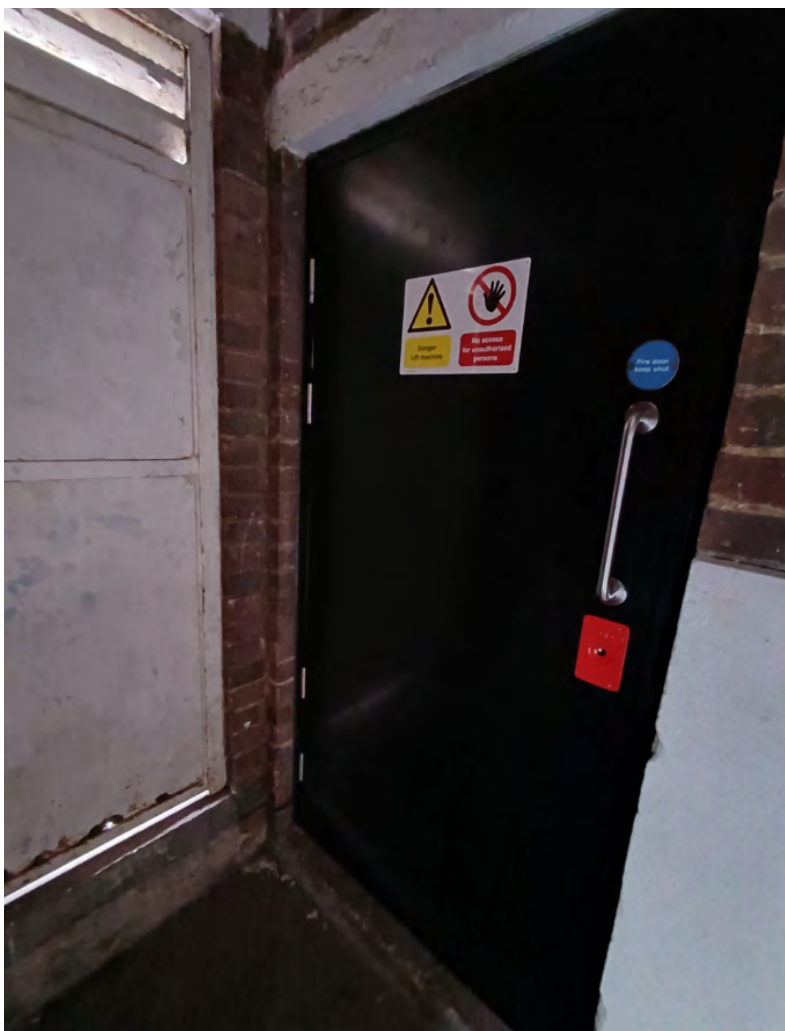
Lift Motor Room Fire Door at Hollisfield.
