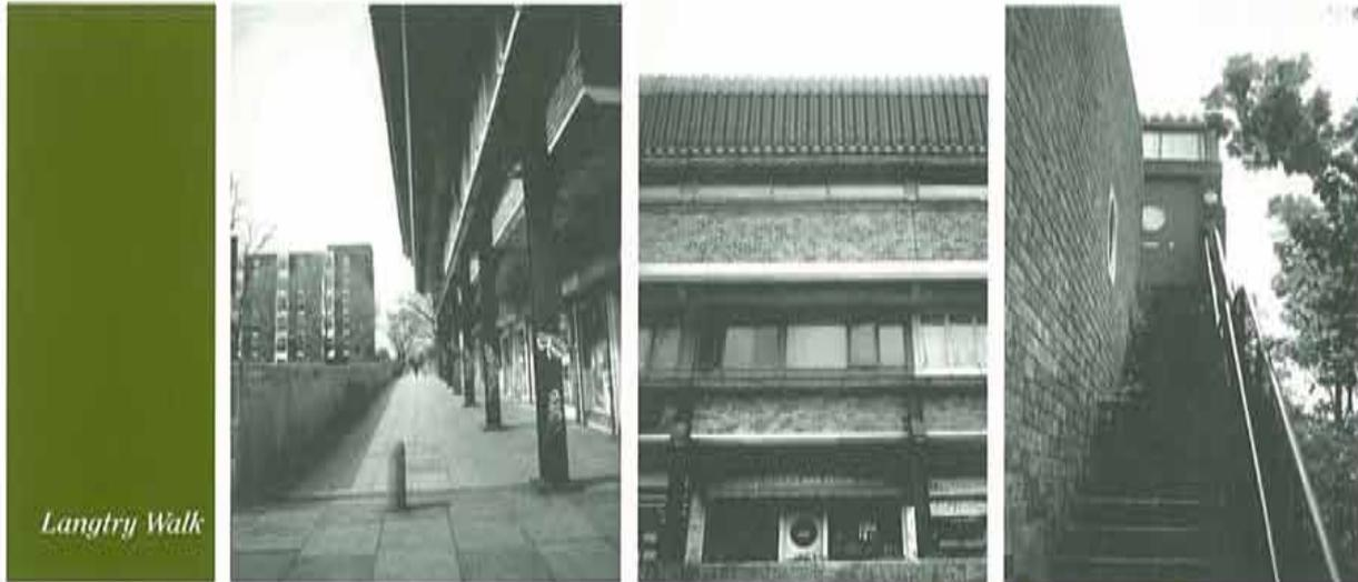
colonnade of steel stanchions supports residential units at first floor. These are **Nos.1-8 Langtry Walk**. At second floor level and to the rear of first floor level are two banks of workshops roofed over with metal to a curved profile, **Nos.61-83 Loudoun Road**, accessed from steps on Loudoun Road. A sunken service yard entered from Loudoun Road occupies the remainder of the site.
