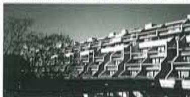
Much of the estate is constructed of fair-faced, white concrete with chamfered arrises. Careful attention was given to the detail and execution of the board-marking and day-work joints. The
